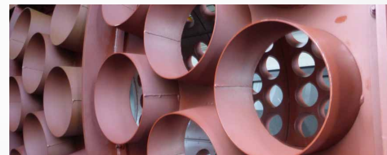
Protection against wrapping by pipe sleeves
